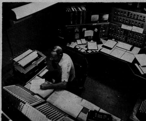
NUCLEAR facilities must be approved by the voters before they can be sited in Montana. Pictured is a control center for computerized surveillance of underground leaks at the waste storage site in Idaho.
