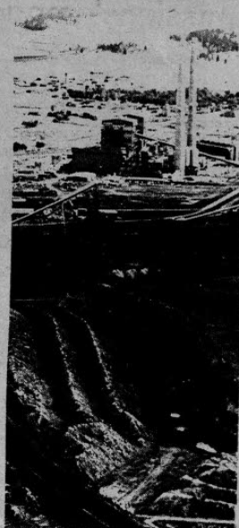
Photo courtesy of EPA RECLAMATION OF COAL STRIP MINES near coal-fired power plants may be stymied by sulfur dioxide emissions' effects on vegetation. Pictured is the Western Energy mine near Colstrip units 1 and 2 in southeastern Montana.
