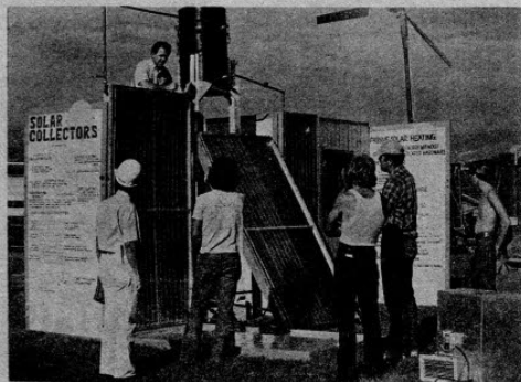
BOTH HOME-BUILT AND COMMERCIAL solar hardware are on display at the New Western Energy Show. Shown here is a home-built solar water heating system.
