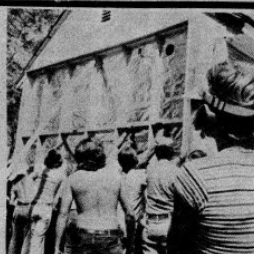
MANY HANDS made mounting the eight by twelve foot solar collector built for the Behring home in Greeley, Colo., light work. In the upper right hand corner is the hot air inlet to the house, and to its right, the thermostat. A black, metal absorber plate and a fiberglass cover were later added to the assembly. Photo by Joy Coombs
