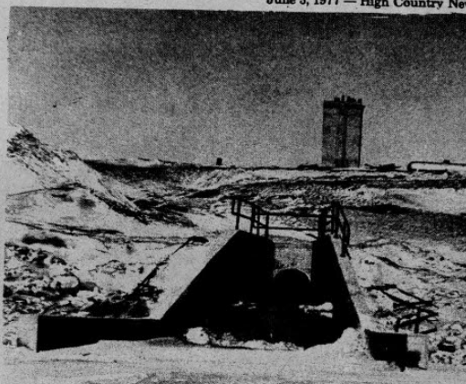
POPLAR RIVER DAM. Saskatchewan Power Co. built this dam, expecting it to fill in three years. No spillways had been built. Within three days after water started flowing into it, it was full, throwing downstream residents into a panic. A sudden change in weather got them through the crisis, and this spillway was added.
