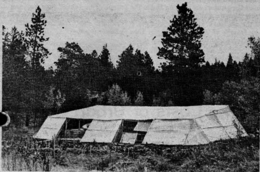
VETERAN. The solar heated greenhouse shown here is Lillywhite's own, a veteran of nine year's production. While this one is leaky, made out of pine poles, plastic, and a fiberglass roof, Lillywhite's more recent designs are nearly airtight. He generally recommends an insulated slab foundation, 2 x 6 construction in the walls, an R-19 in the north, east, and west walls, and an R-30 in the ceiling. The clear, south-facing wall is covered with fiberglass and polyethylene.
