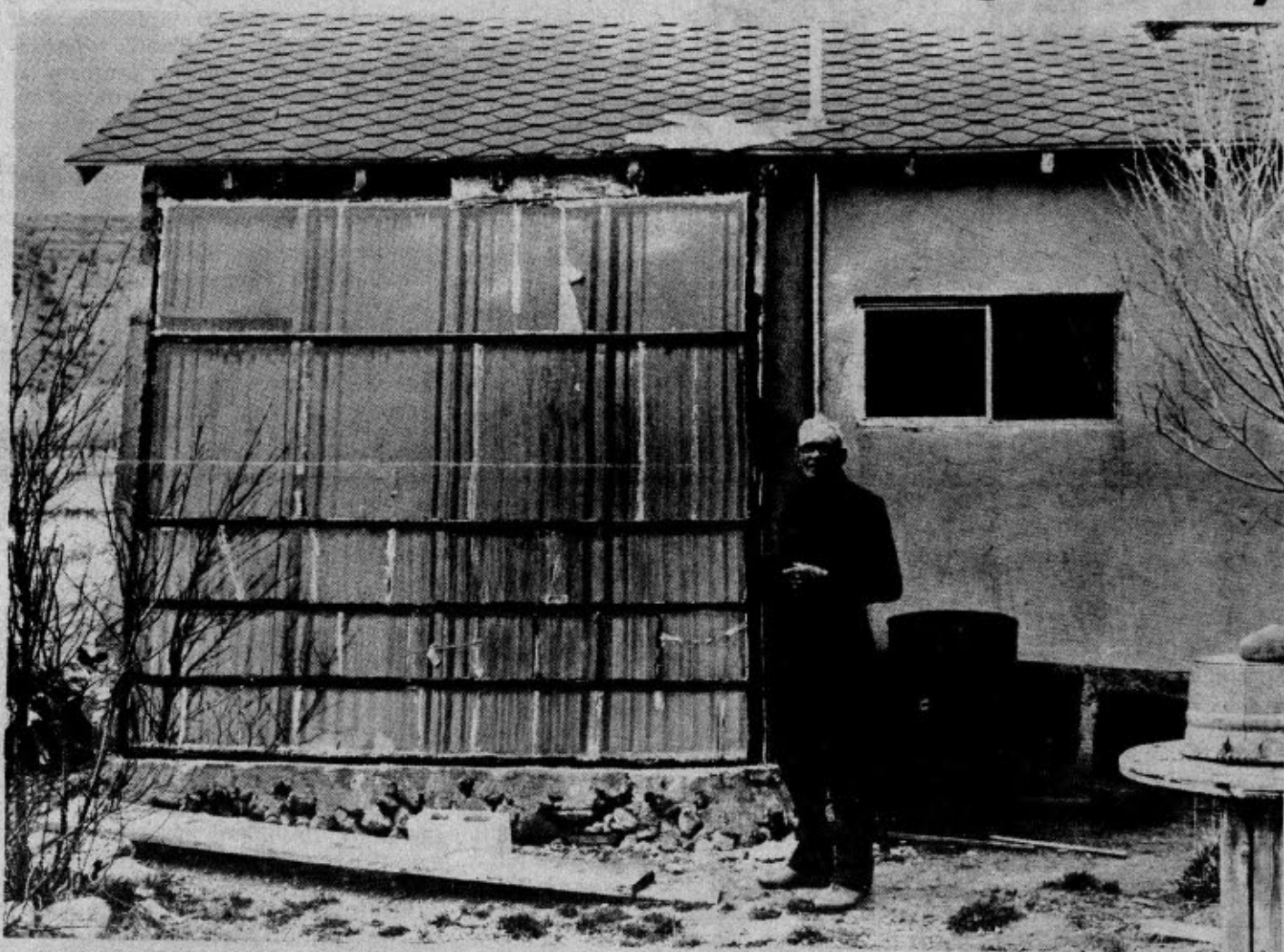
PHARMACIST STIRRING UP NEW STORAGE SYSTEM. Paul Wise, a retired pharmacist, is experimenting to find an improved storage material for the heat he collects in his home-made solar collector. The system,
