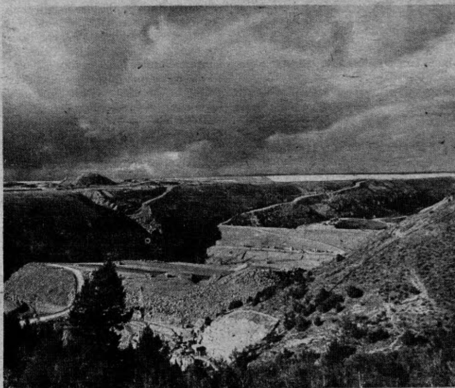
TETON DAM under construction on the Teton River in eastern Idaho. When the dam broke, there were millions of dollars of damage and seven human lives were lost. Photo by David Sumner.
