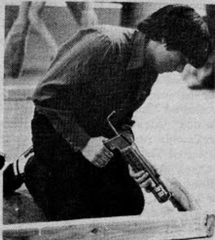
SEALING THE BOX with caulking compound.
