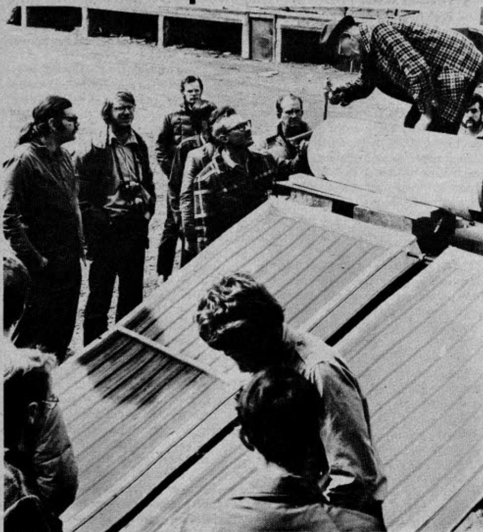
CONNECTING WATER TANK TO COLLECTORS. The prospects for immediate success looked dim that day in Billings because the sky was so overcast.
