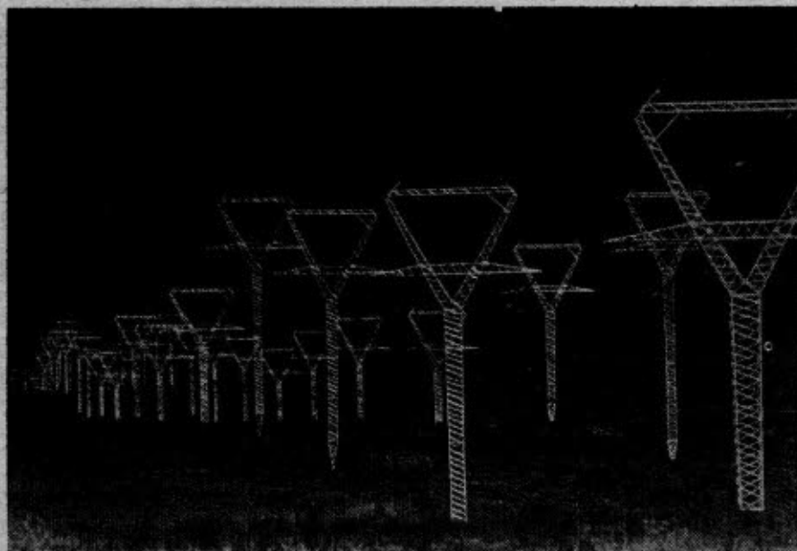
Two of the three 345 kv lines from the Jim Bridger coal-fired generating plant near Rock Springs, Wyo. Photo by Gowen Green.
