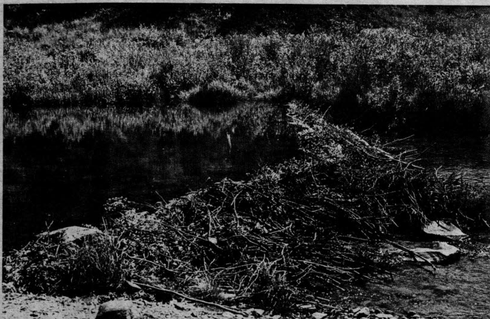
The dam is often curved with the flow of the stream for added strength.
