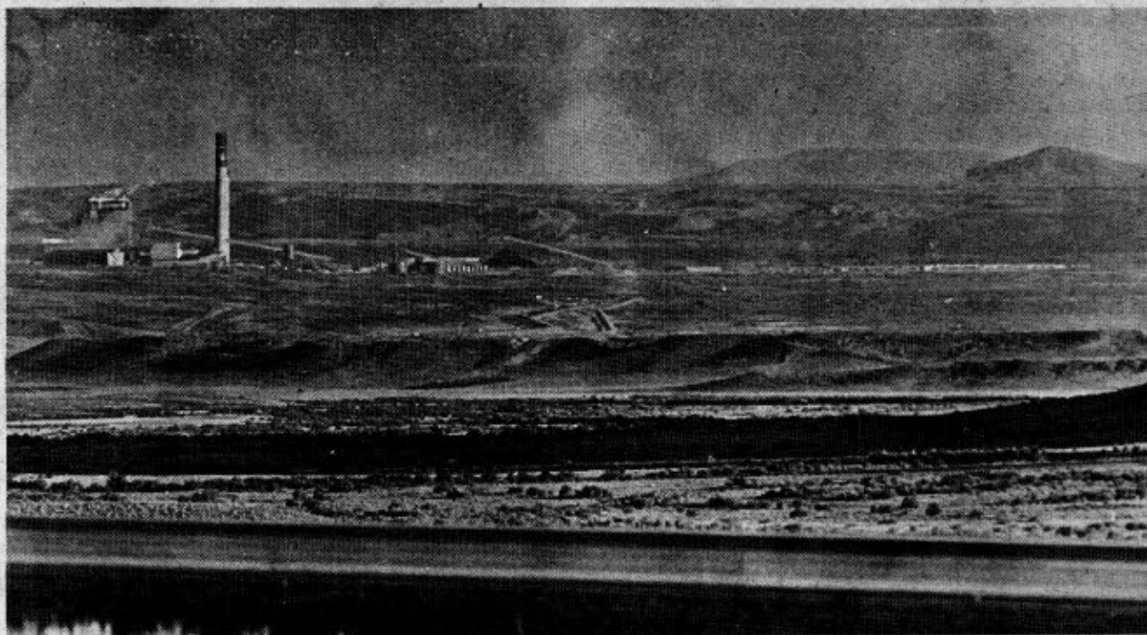
The entire Jim Bridger complex is visible from the highway. From left to right: the boiler and cooling tower, precipitator, three stacks (almost in line), coal conveyors and storage yard (not full yet), and trailers in the construction camp. The switchyard is also visible from I-80 but is off the left side of the picture.
