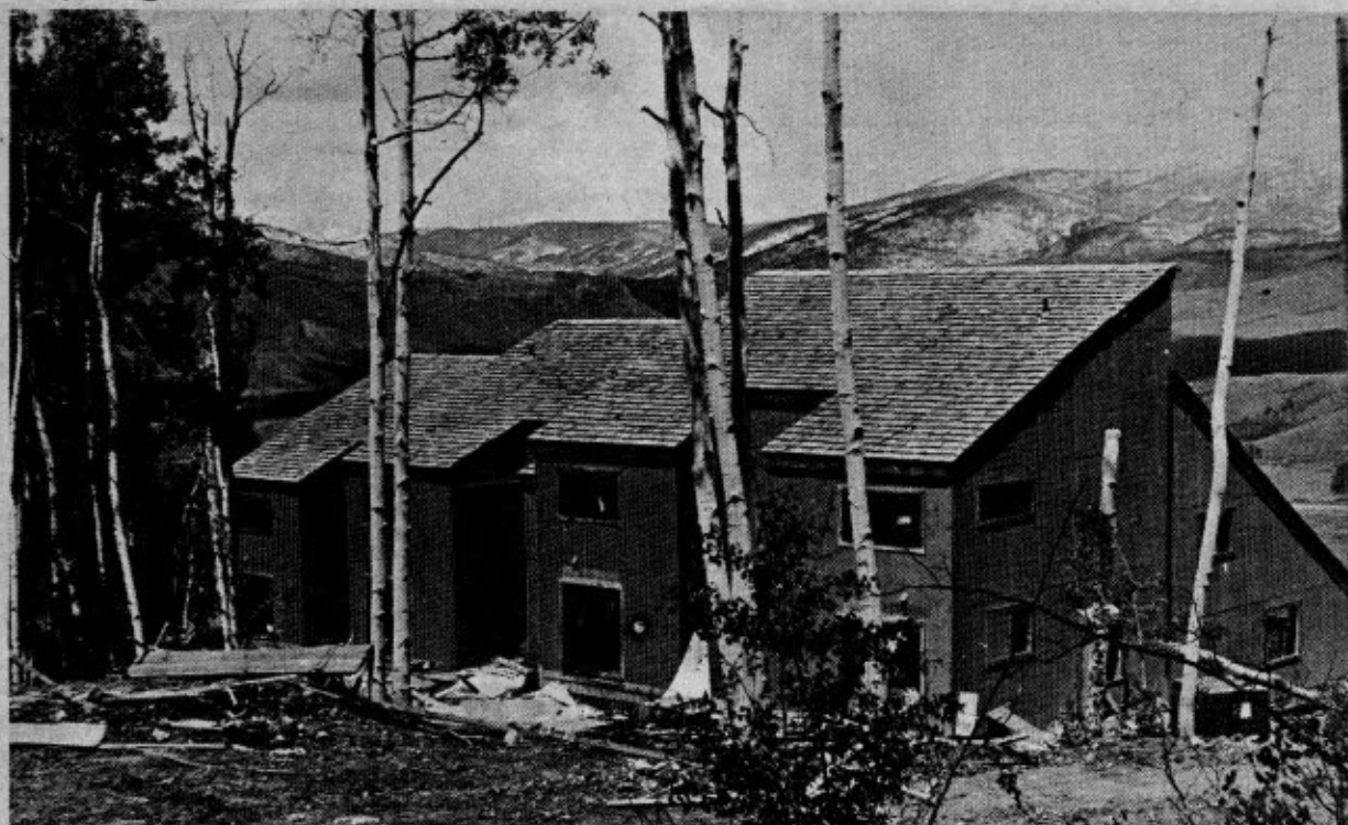
The Stagecoach development near Steamboat Springs is one of Colorado's newest ghost towns. With construction 30% complete, the project's developer, the Woodmoor Corp., declared bankruptcy early this year. The recreational community was planned to bring over 30,000 vacationers to Routt County (population 7,000).
