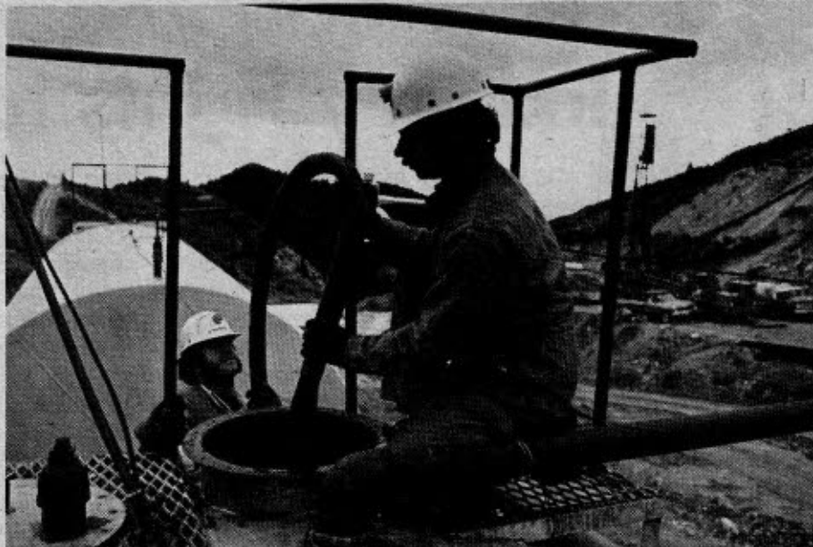
Occidental technicians pump recovered shale oil from a sump in the retort into 26,000 gallon tanks on top of the mountain. In actual production, all tankage will be underground.
