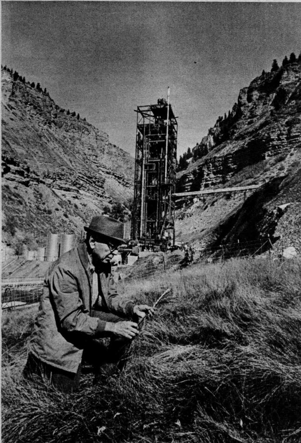
A revegetation plot at the Colony Development Operation pilot plant in Parachute Creek Canyon near Grand Valley, Colo. Once the canyons are filled to the brim with oil shale wastes, the companies hope to establish plant cover to stabilize the wastes and return them to a productive state. The tower in the background is Colony's retort which heats the crushed oil shale and drives the petroleum from the rock.
