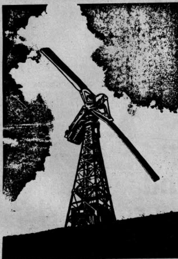
The Smith-Putnam wind turbine atop 2,000 foot Grandpa's Knob near Rutland, Vt. Each eight ton blade rotated at a maximum speed of 29 revolutions per minute to produce up to 1500 kilowatts of alternating current. This wind turbine was the largest one ever constructed and was the first one to feed power routinely into commercial power lines. Structural cracks in one blade caused it to fly off on March 26, 1945. The blade sailed 750 feet down the mountain and the machine was never repaired. The project was abandoned as a $1,250,000 experiment.
