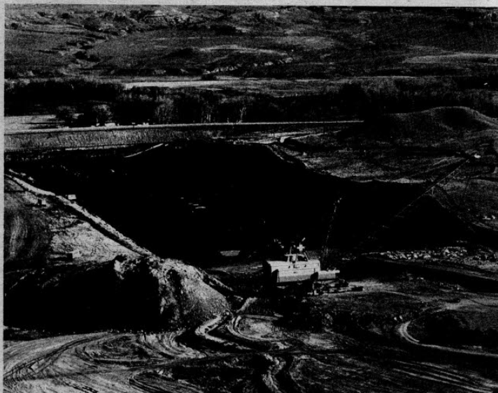
Decker Coal Co. is a joint venture between the large construction firm of Peter Kiewit & Sons and Pacific Power & Light Co. The mine, shown here in the initial stages, is located along the Tongue River just north of the Montana-Wyoming state line. The coal seam is 52 feet thick, just beneath the surface. Unit trains will haul some four million tons from here to Havanna, Ill., where it will be loaded on barges for shipment to Commonwealth Edison in Chicago. The mine is equipped to handle a much larger tonnage.
