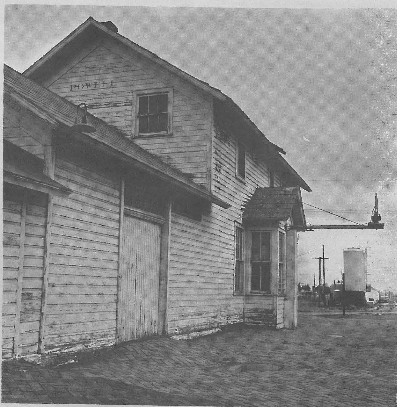
Powell, Wyo. Dilapidated stations mark most western small towns.
