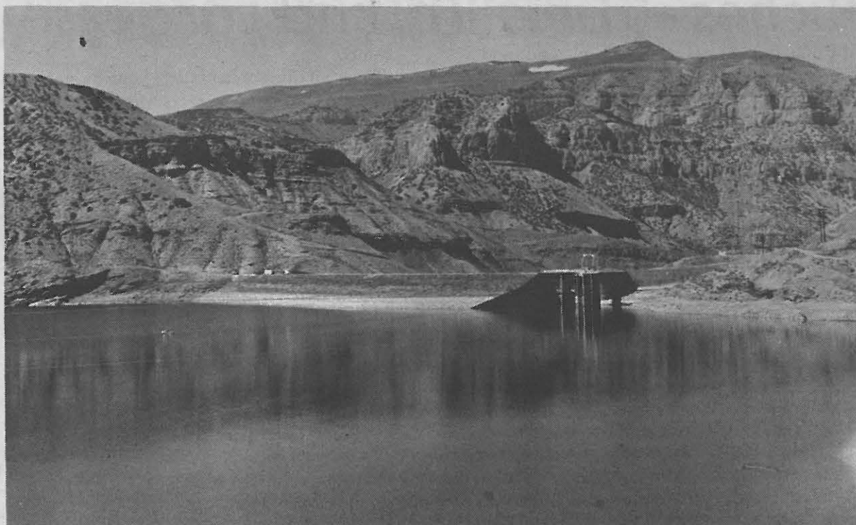
Boysen Reservoir on the Wind River near Riverton, in central Wyoming will supply large amounts of water to the growing energy industry in the Powder River Basin.
