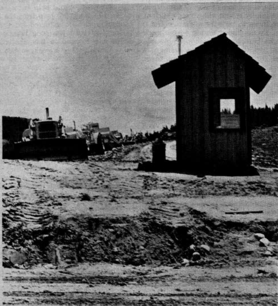
A sign of the times on the western scene — a developer's sales shack and a row of bulldozers ready to go to work on the mountain landscape. Literally millions of acres of beautiful western lands are being remade in the mold of the developer's image. Without effective legislation, land planners and citizens alike are frustrated in their efforts to protect the land.
