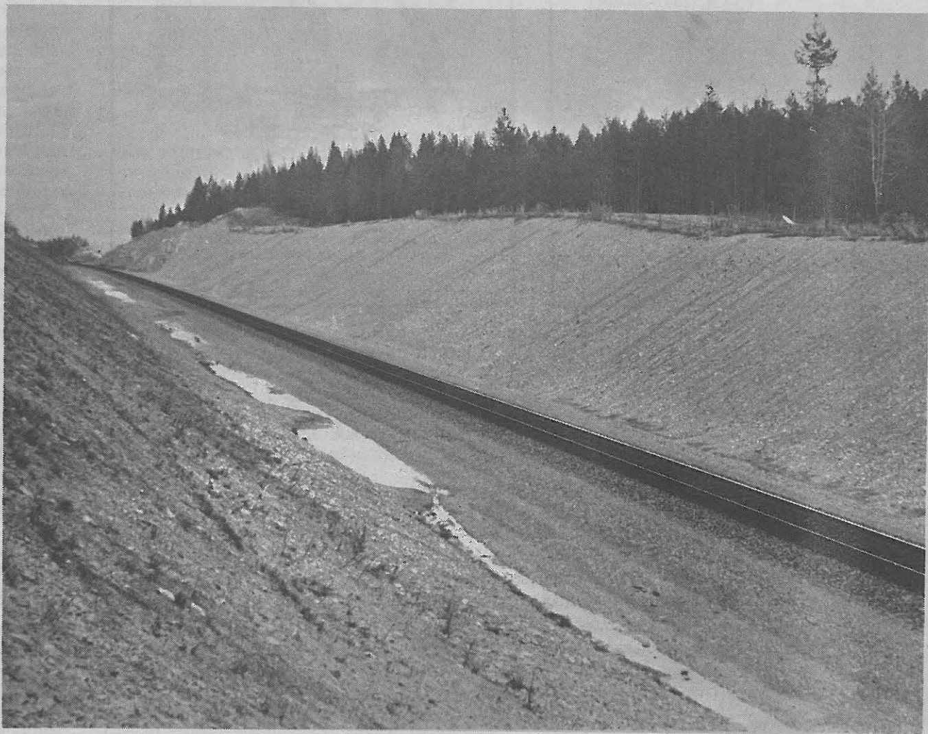
This scene is typical of many of the deep cuts made along the relocated Burlington Northern line. The material from this cut was stacked in a pile a half-mile long and several hundred yards wide. The pile is to be revegetated under restoration plans.
