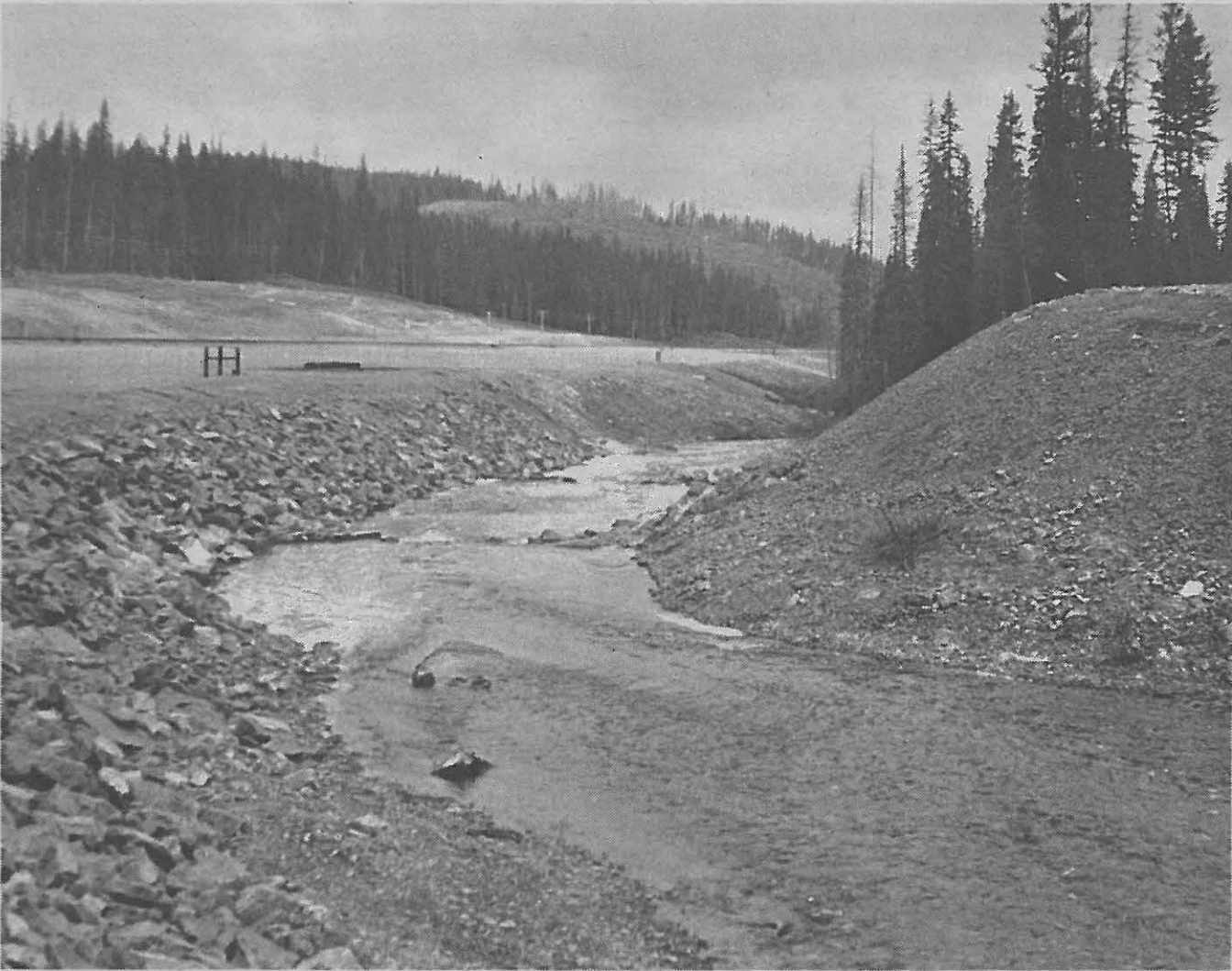
Channelized Fortine Creek, looking north, from the north portal of the Trego Tunnel on the Burlington Northern Railroad. Relocation was necessary because of the construction of Libby Dam. (Yes, that's a clearcut in the background.)
