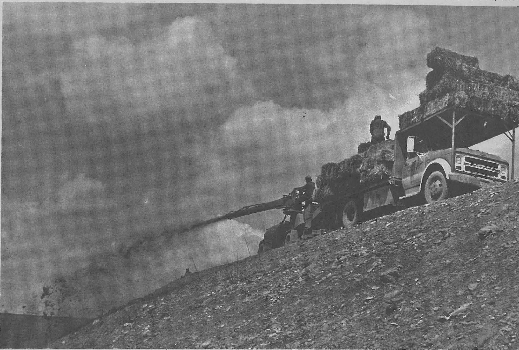
Mulching and seeding of a road grade at the Cripple Creek crossing of the newly relocated railroad line.
