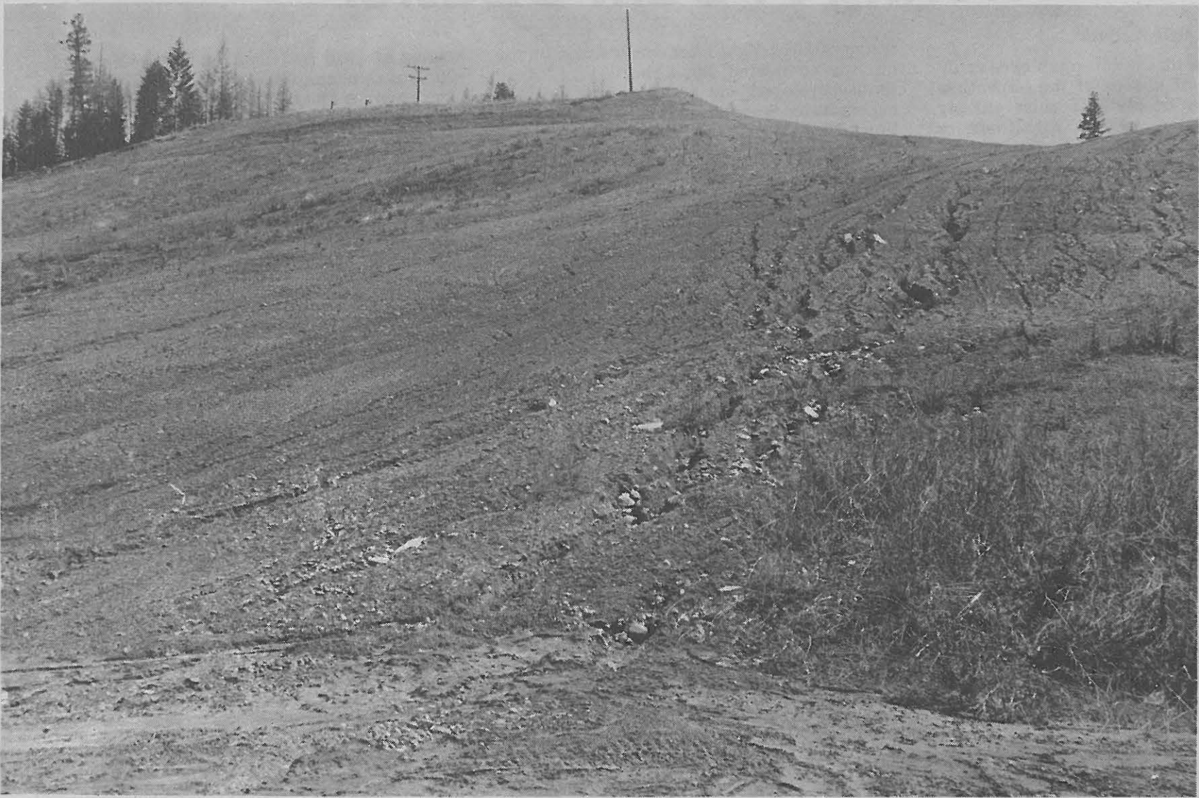
A vast area of gully erosion brought about by the relocation of the Burlington Northern Railroad. The fence halfway up the slope denotes the division of responsibility between the Corps of Engineers and the Burlington Northern. The Corps will contract restoration work on top of the hill (out of sight) for about a quarter of a mile. BN is responsible for stopping erosion in the foreground, which has gone unchecked for two years.
