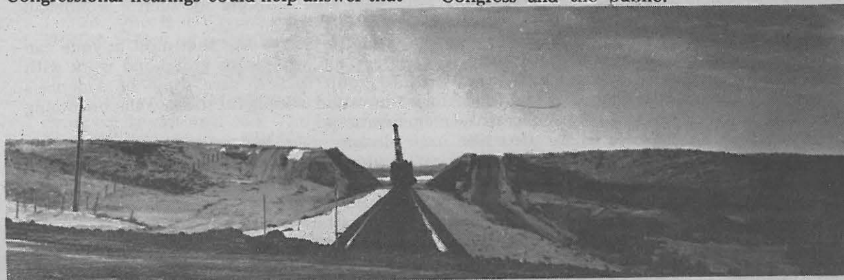
A new railroad spur being built to the strip mine now operating at Decker, Montana.
