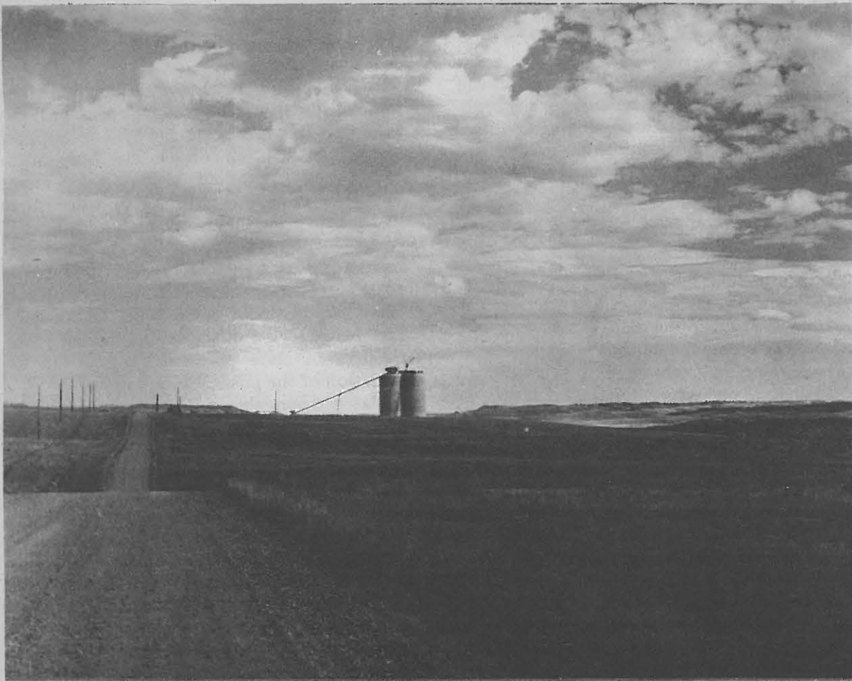
The huge, twin silos of Ayrshire Coal Co. (a subsidiary of American Climax Molybdenum) rear above the prairie in Wyoming's Powder River Basin. Coal from a strip mine (at right) will go to feed the power plants at some distant location in the east. An 18-mile spur from the Burlington Northern Railroad was built to haul the coal away. Additional developments such as this will lead to the strip mining of thousands of acres of this rural land.
