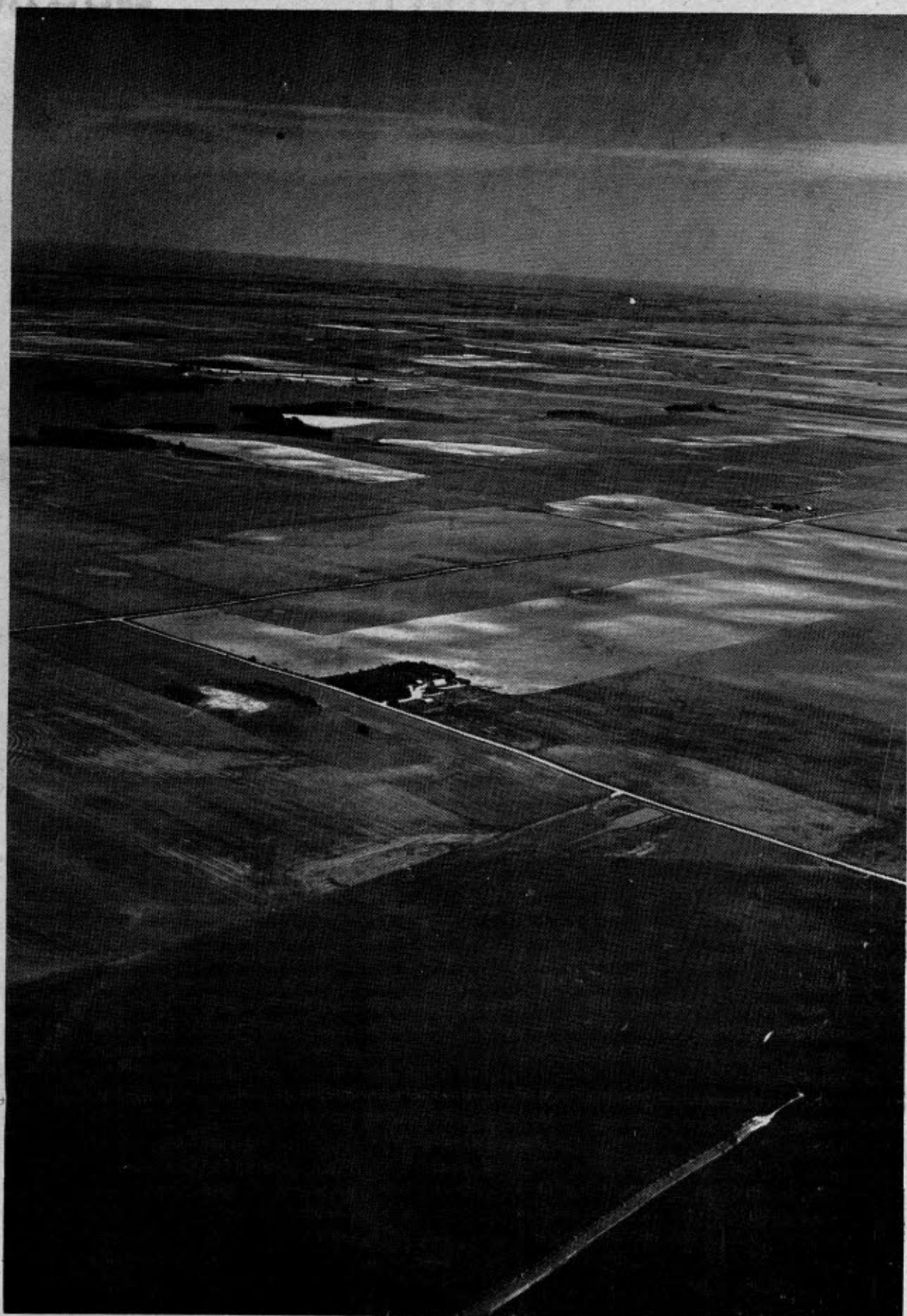
A $180-million, 600-megawatt power plant will occupy this productive Nebraska farm land if the Public Power Review Board authorizes the project. The ash pit to accommodate some 700 tons of ash per day will occupy one square mile on land centered around the farmstead in the foreground. The plant will be located near the farmstead at right, center. The present air quality is demonstrated in this aerial photo.
