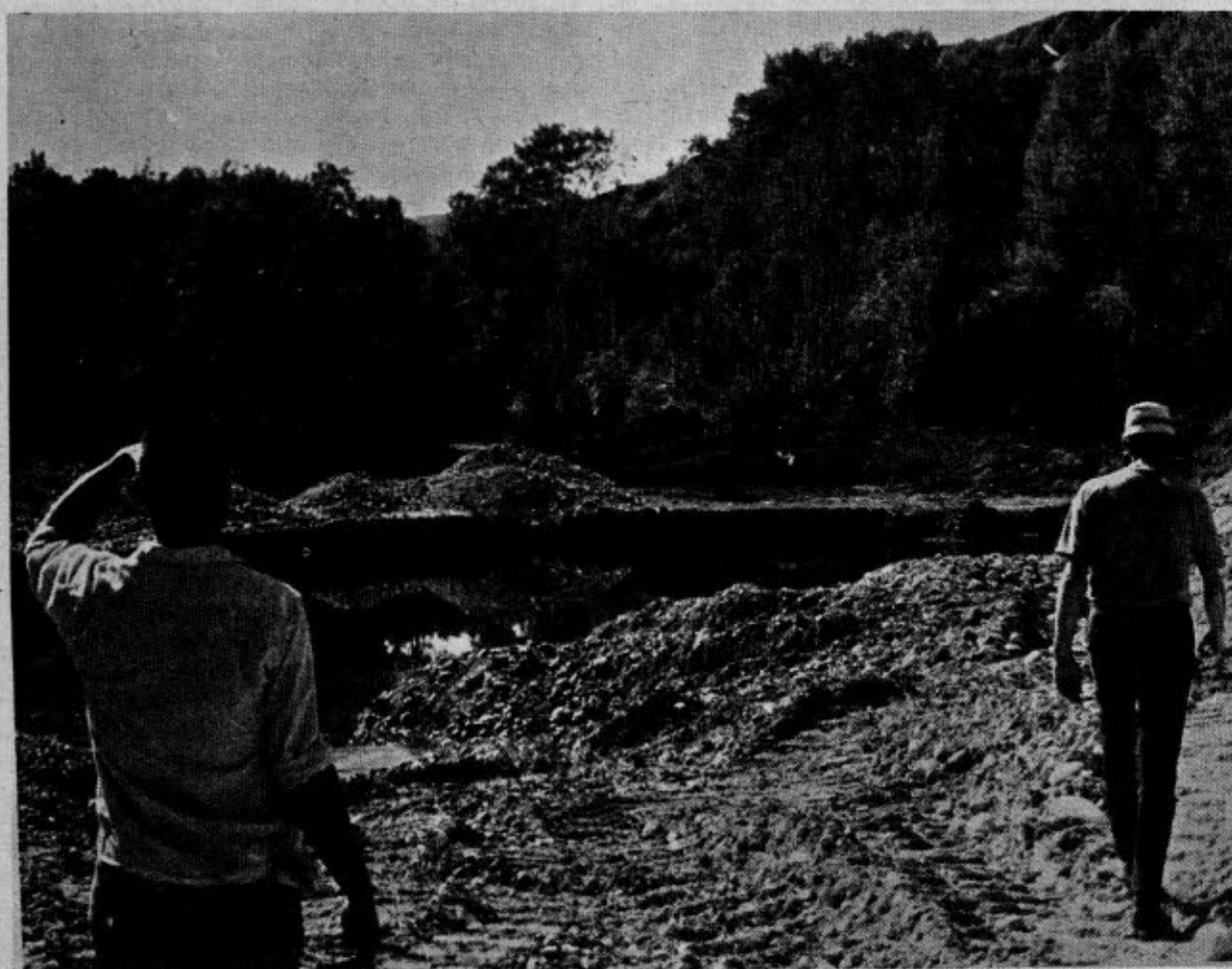
On site in the area of the Lower Teton Dam in Idaho. The Bureau of Reclamation dug seven one-acre test holes to provide for inspection of gravel. Preliminary construction work is now underway on the controversial project.
