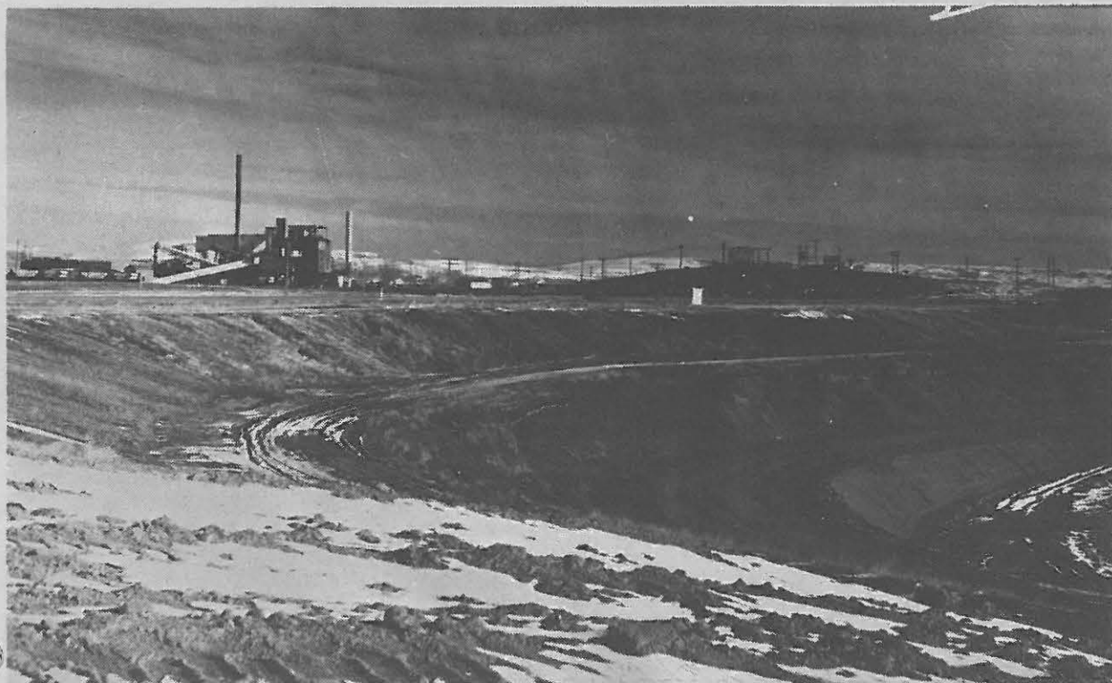
The first of many mine-mouth steam-generating electric plants in Wyoming and Montana's Powder River Basin is located six miles east of Gillette, Wyoming. This relatively small plant of 27,600 kilowatts uses air-cooled condensers. Plans have already been announced for an expansion of the plant to a 200,000 kilowatt capacity. That facility is to be in operation by 1976.
