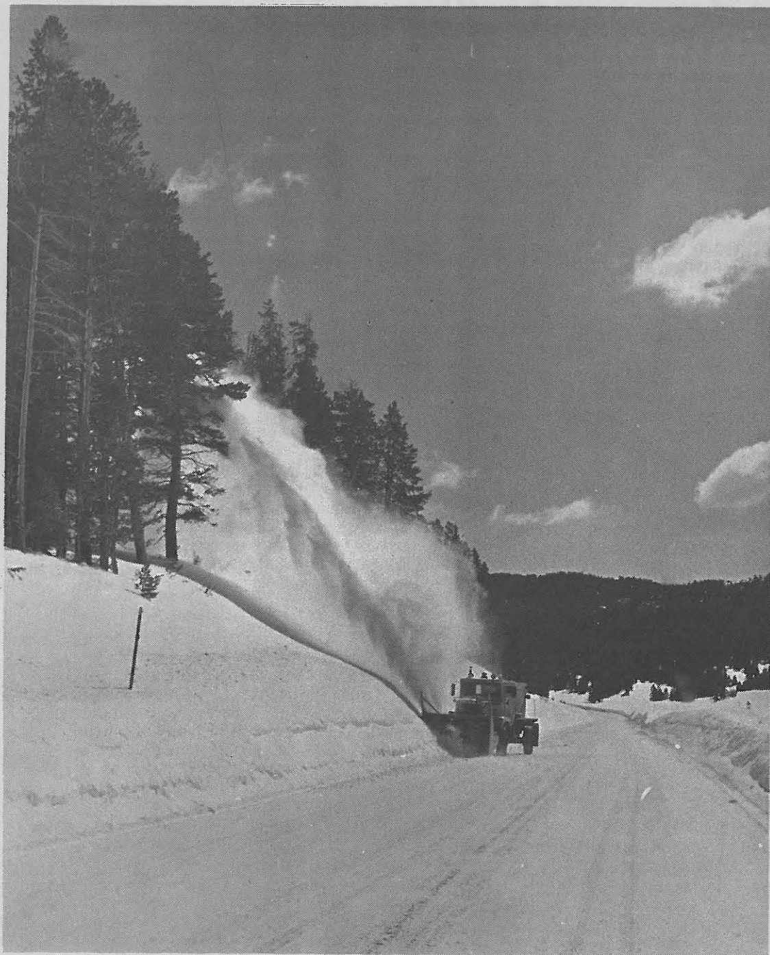
A rotary snowplow clears the highway on Togwotee Pass between Dubois and Jackson, Wyoming. Heavy snows in the mountainous regions of the West make highway maintenance difficult. Yellowstone National Park highways should open on Schedule, May 1, unless other spring storms interfere.
