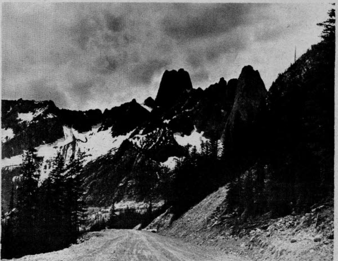
A typical scene along the North Cross-State Highway now under construction through the North Cascades National Park in Washington State.
