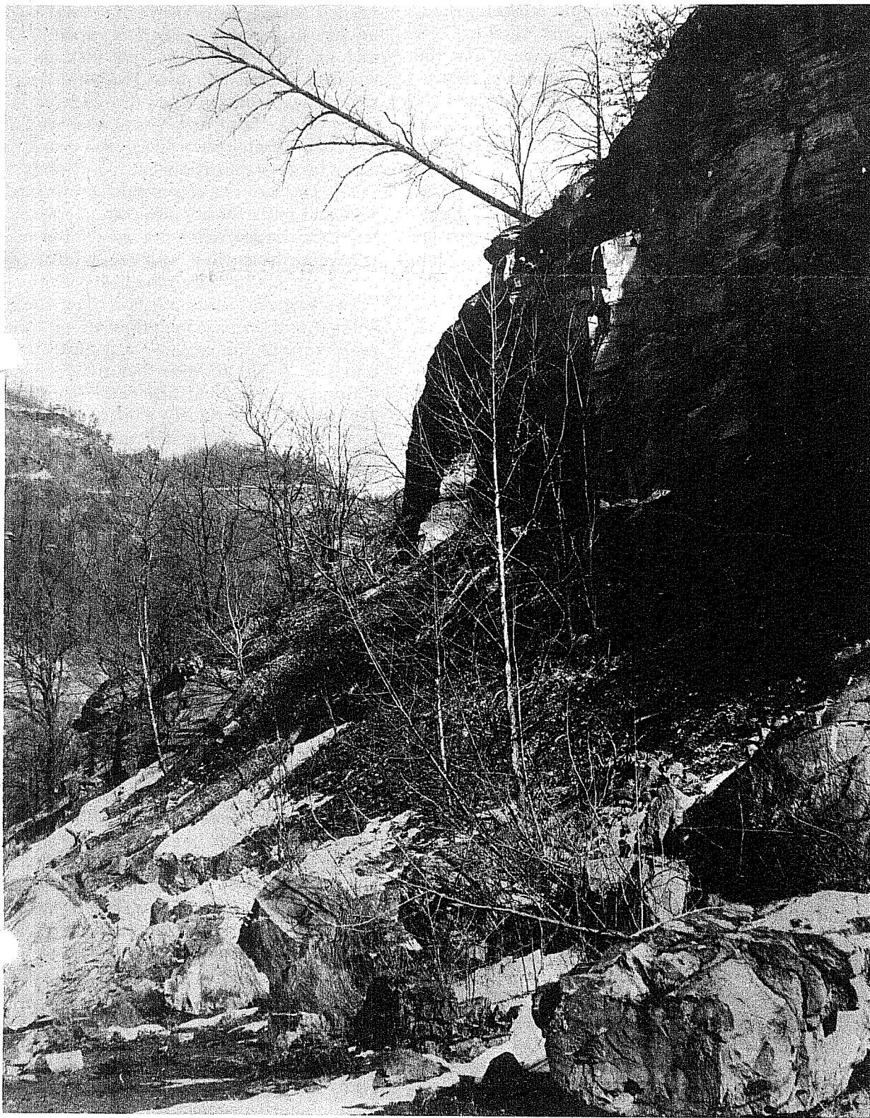
West Virginia has already been hit by the destructive forces of strip mining. Here a highwall and the area just under it have begun to recover after ten years. But the highwall keeps breaking off since it was shattered years ago by blasting which preceded the bulldozer.
